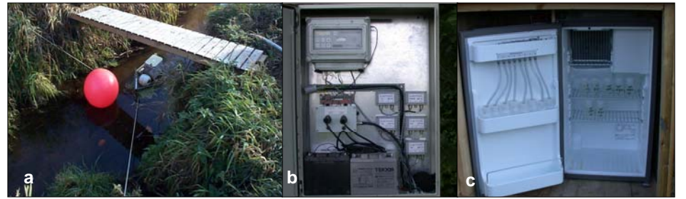
Fig. 4: Instruments of the automatic sampling stations; a. sensors in the stream; b. sensor amplifiers and data logger; c. water sampling and cooling (design: Dr. W. Schäfer, Ambio-Tec, Palzing)
